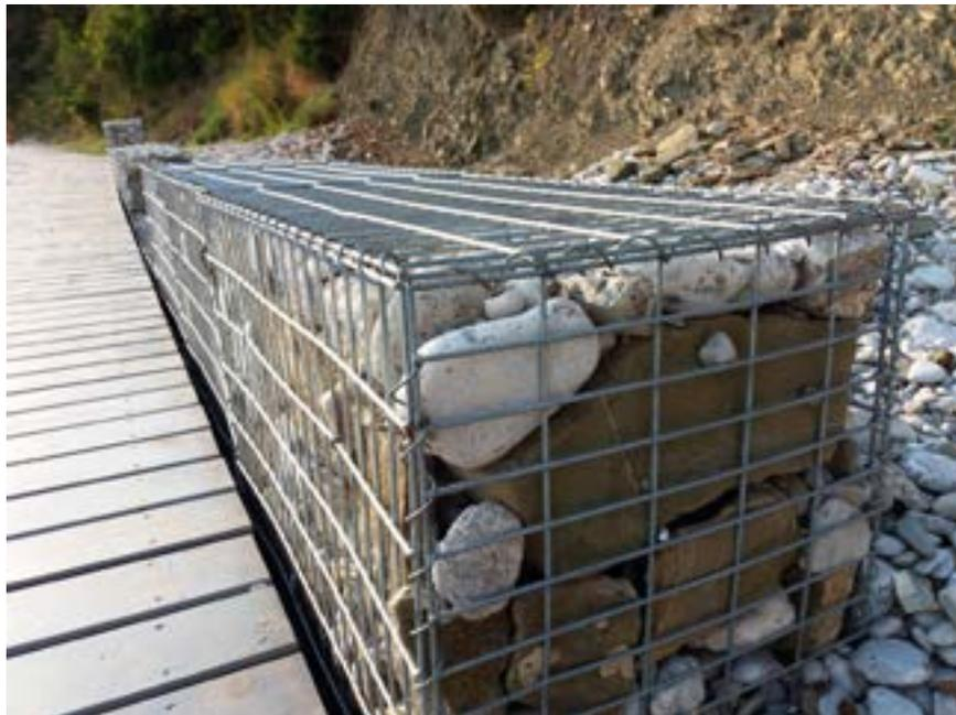
**Fig 14: Gabions at base of cliff**
