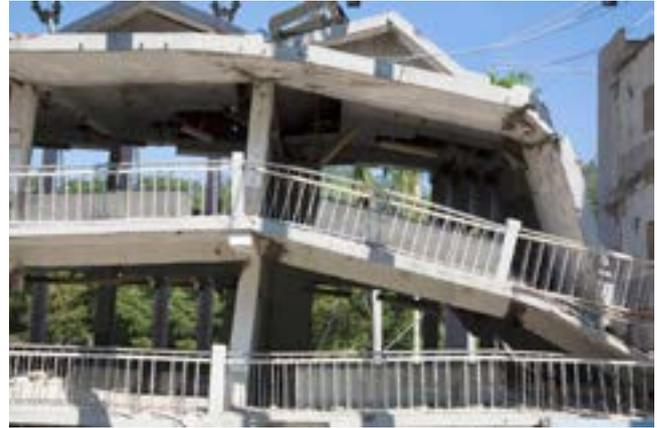
**Fig 2: Damage to a building caused by an earthquake**
