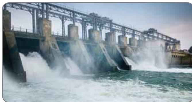
Hydroelectric power stations use kinetic energy from moving water. The water normally comes from behind a dam built across a river valley. The water high up behind the dam acts as a store of potential energy. This is transferred to kinetic energy as the water passes down through the inside of the dam. The moving water directly **drives turbine blades which in turn drive electrical generators, which are normally housed inside the dam.**
