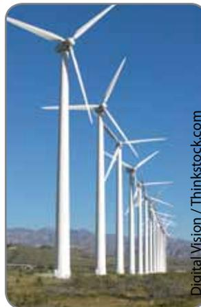
Wind power turbines have blades mounted on a tall tower. The blades are connected to a housing that contains gears linked to a generator. As the wind blows, kinetic energy from the wind is transferred directly to the blades, which rotate driving a gear system which in turn drives a generator. Several wind turbines are normally grouped together in windy locations to
