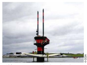
A tidal stream generator such as the one located on Strangford Lough operates using what are essentially underwater turbines. These use the energy provided by fast
